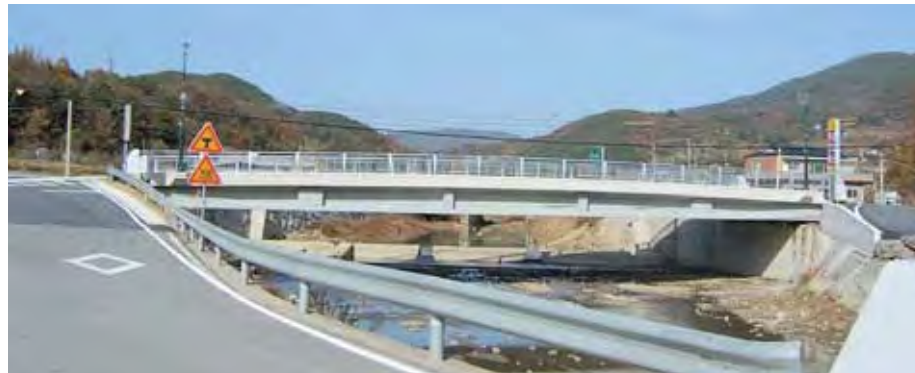
CHA HANG BRIDGE (韓国:SPC単純桁橋)
